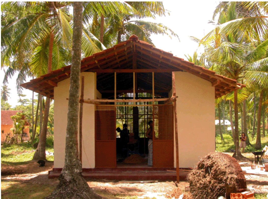
Figura 12- Fachada Safe (R) House
